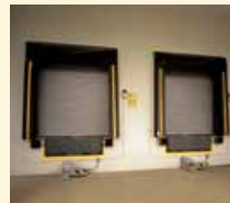
Rolling Service Doors
